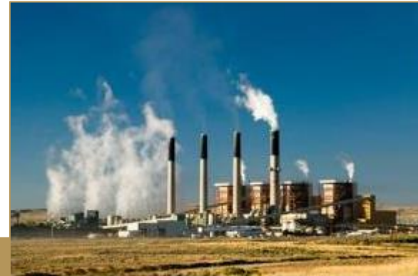
Cochise Power Plant, Arizona
