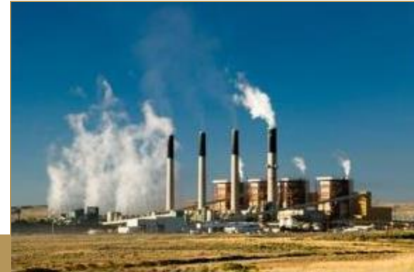
Cochise Power Plant, Arizona
