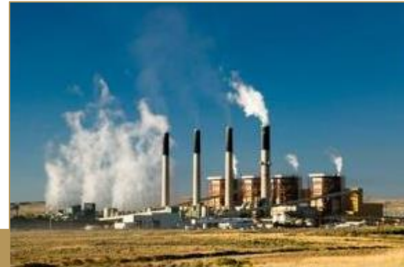
Cochise Power Plant, Arizona
