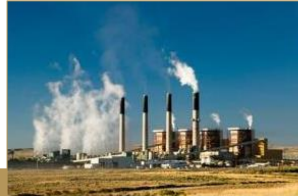
Cochise Power Plant, Arizona
