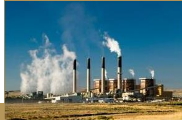
Cochise Power Plant, Arizona
