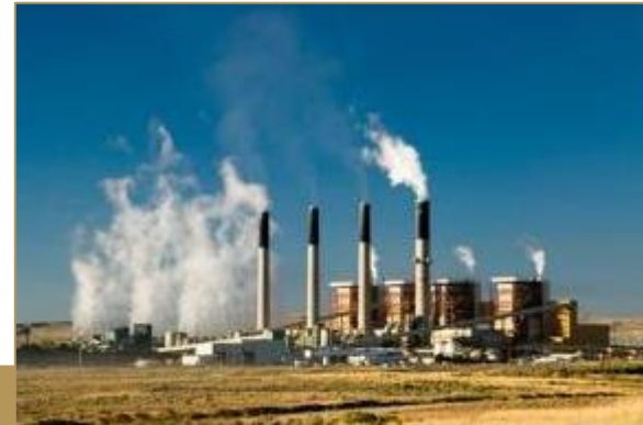
Cochise Power Plant, Arizona
