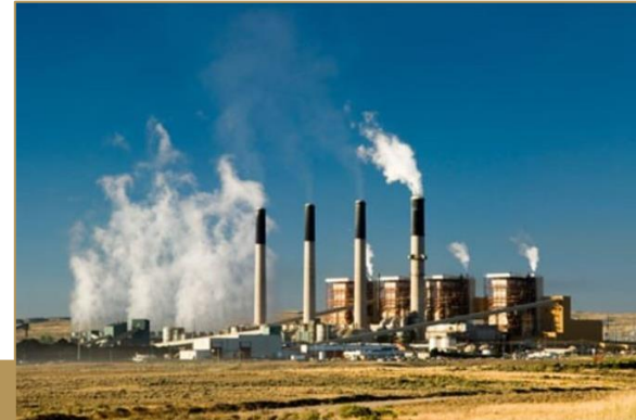
Cochise Power Plant, Arizona
