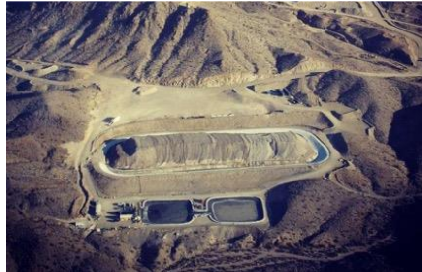
International Vertex's Moss Mine in Arizona
